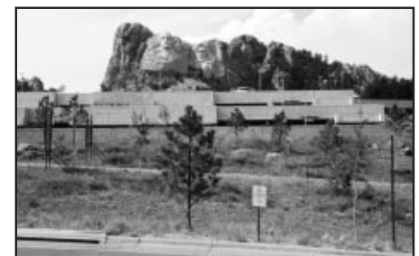
The new National Park Service parking structure, with vegetative buffer (in a few years), at heavily visited Mt. Rushmore. Entrance to the National Monument is free, but it costs $8 to park here. A free lot is available further away.
