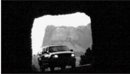
The roadway improvements suggest a real attention to detail to best showcase the natural (and human-made) environment. Mt. Rushmore can be seen in the background.
