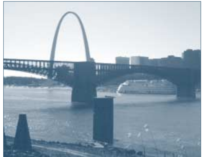
In 1874 James Buchanan Eads completed the Eads Bridge, which is located along the Historic National Road in Illinois. Listed on the National Register of Historic Places, the Eads Bridge was the first across the Mississippi River below the Missouri River, the first to rely heavily on steel, and the first to use cantilever construction. Today the Eads Bridge is open to vehicle traffic during the week and open to pedestrians and bicycles on weekends. Credit: Photo by Lyle Kruger
