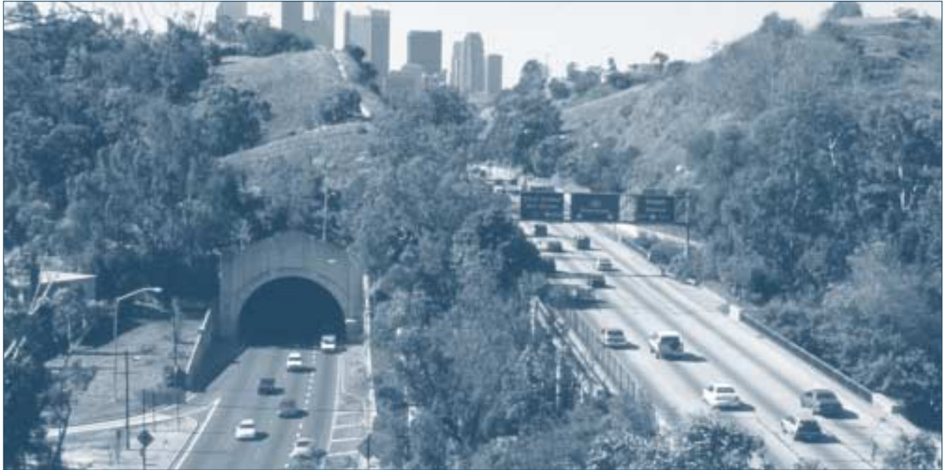
This view of the Arroyo Seco Parkway from atop Elysian Park showcases the Figueroa Tunnels and a view of the Los Angeles skyline. Credit: Photo by Steve Devorkin of Caltrans
