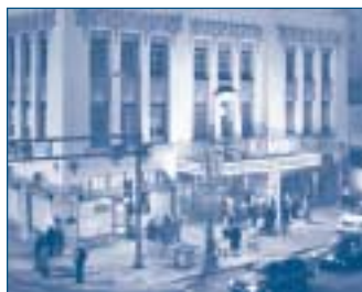
Built in 1927, the KiMo Theatre features restored Pueblo Deco architecture, which fused the spirit of the Indian cultures of the Southwest with the exuberance of America during the roaring twenties. (Credit: www.marblestreetstudio.com )
