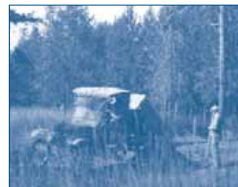
A crew constructs a gravel road near Diamond Lake.
