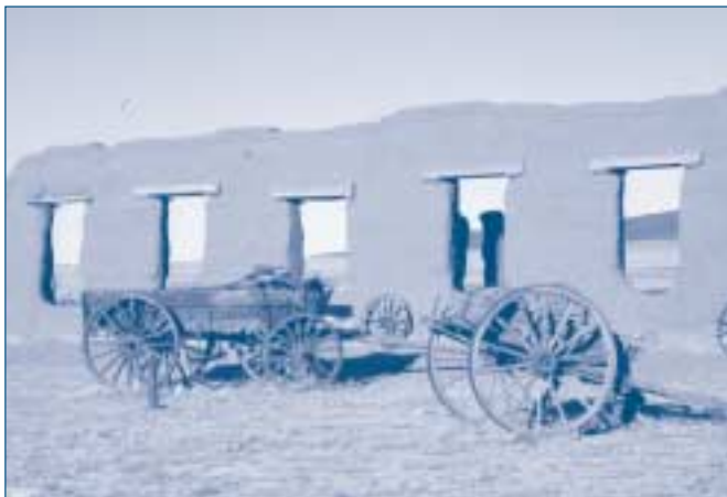
The ruins of Fort Union are an impressive memorial to the men and women who won the West. Stone foundations and adobe walls are remnants of what was once the largest U.S. military installation on the 19th-century southwestern frontier.
