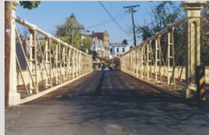
Hunterdon County Bridge, Clinton NJ
